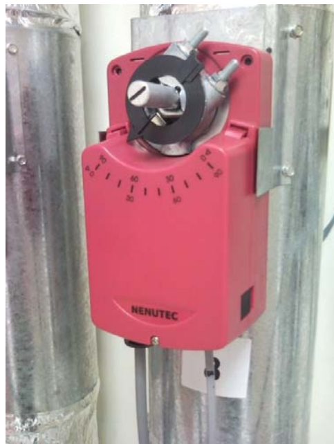
Figure 3.5 A damper actuator which takes an analogue command input
