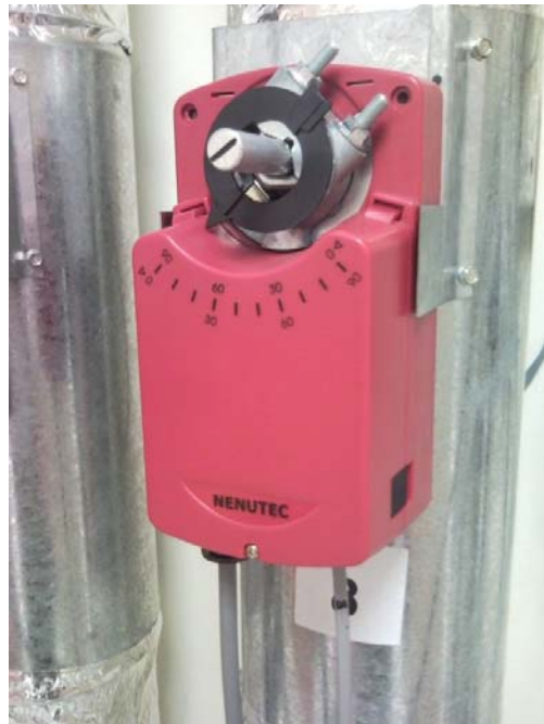
6.4 Motorised damper to regulate airflow
