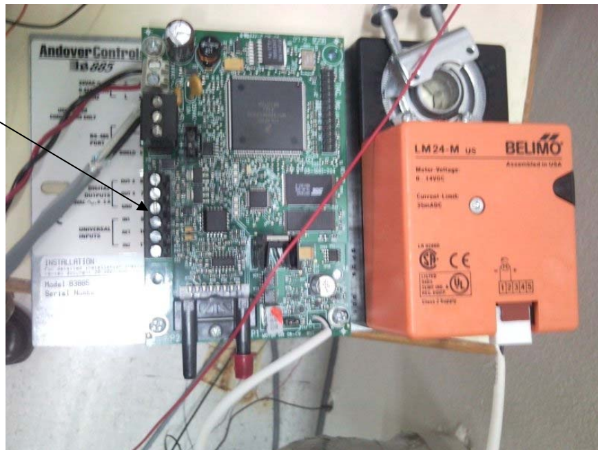
Figure 3.4 A damper actuator which takes a binary command input
